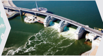
Gangjeong Goryeongbo (weir)
